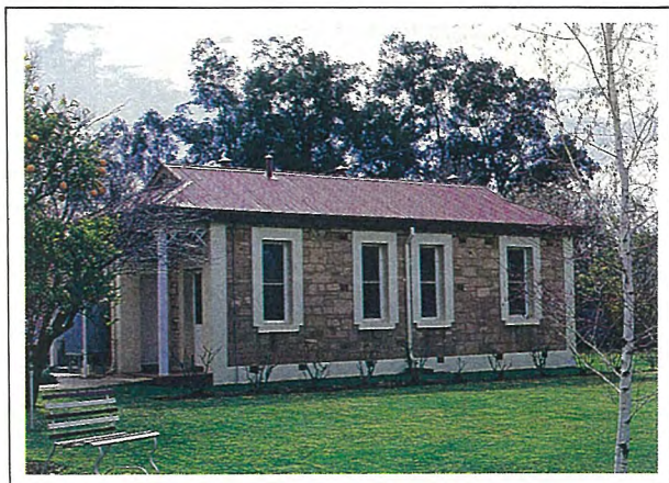
ONE OF THE INTERESTING OUTBUILDINGS
