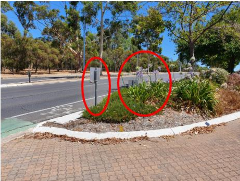
Site 4 westward impeding vegetation and signage:
