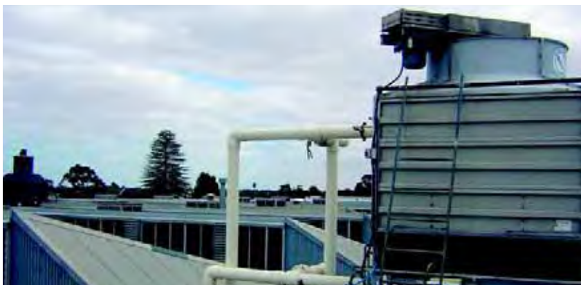
Effective maintenance of cooling towers is necessary to control Legionella
