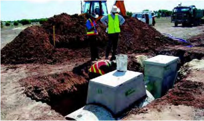
Installation of a waste control system
