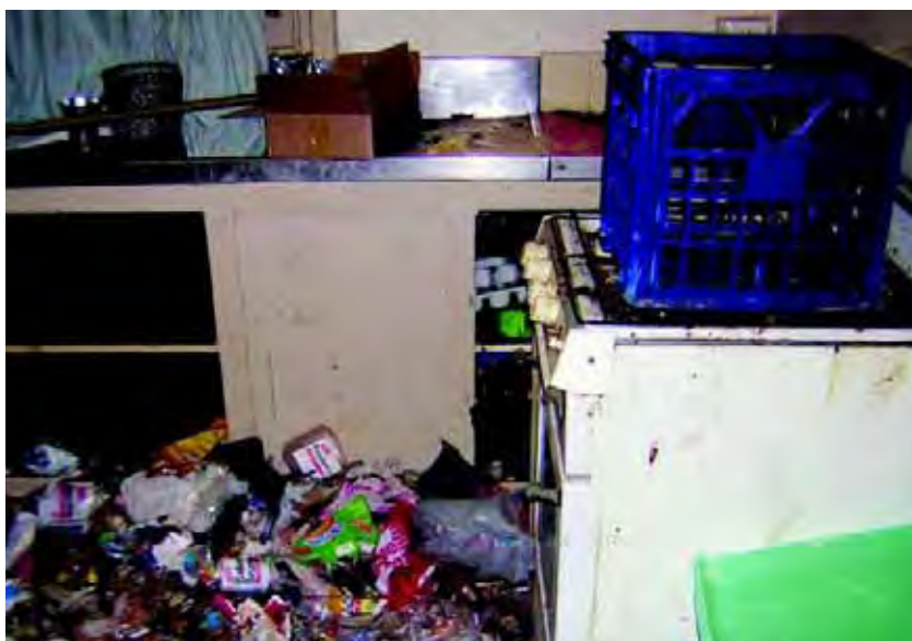
Accumulation of rubbish creating an insanitary condition
