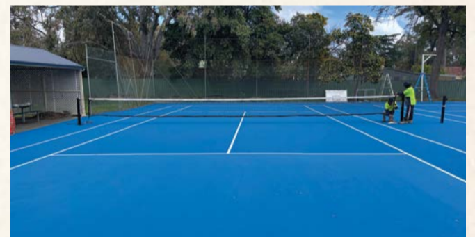
Resurfaced tennis courts at Willow Bend as part of the Ascot Avenue precinct upgrade.
