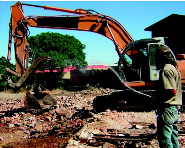
Water used as a dust suppressant on a building site
