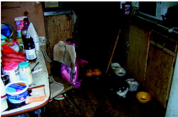
The kitchen of a residential dwelling in an insanitary condition
