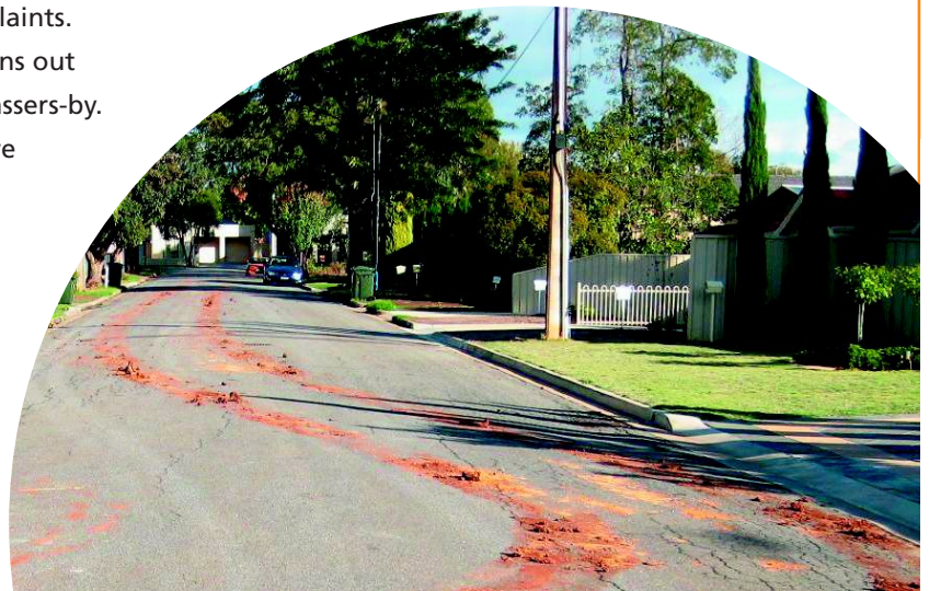
Mud dragged onto the road from a building site
