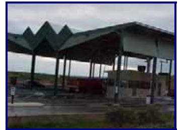
Common Weighbridge for the WWRC
