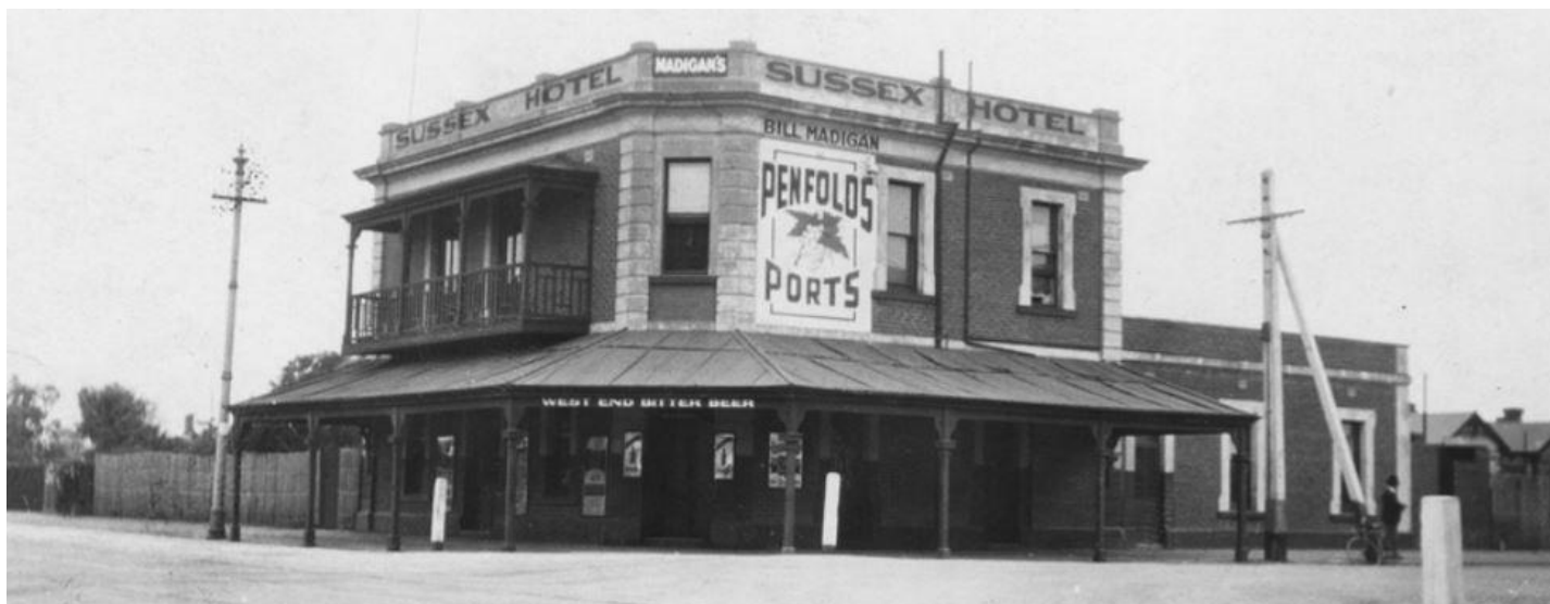
Sussex Hotel, 68 Walkerville Terrace, Walkerville, photographed in approximately 1930 prior to reconstruction works in 1937.
