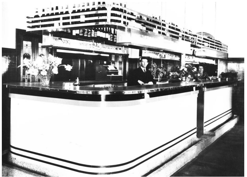
New bar installed at Sussex Hotel during 1937 reconstruction works, photographed shortly after completion.
