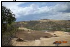
Reprofiled and capped site being covered with mulch
