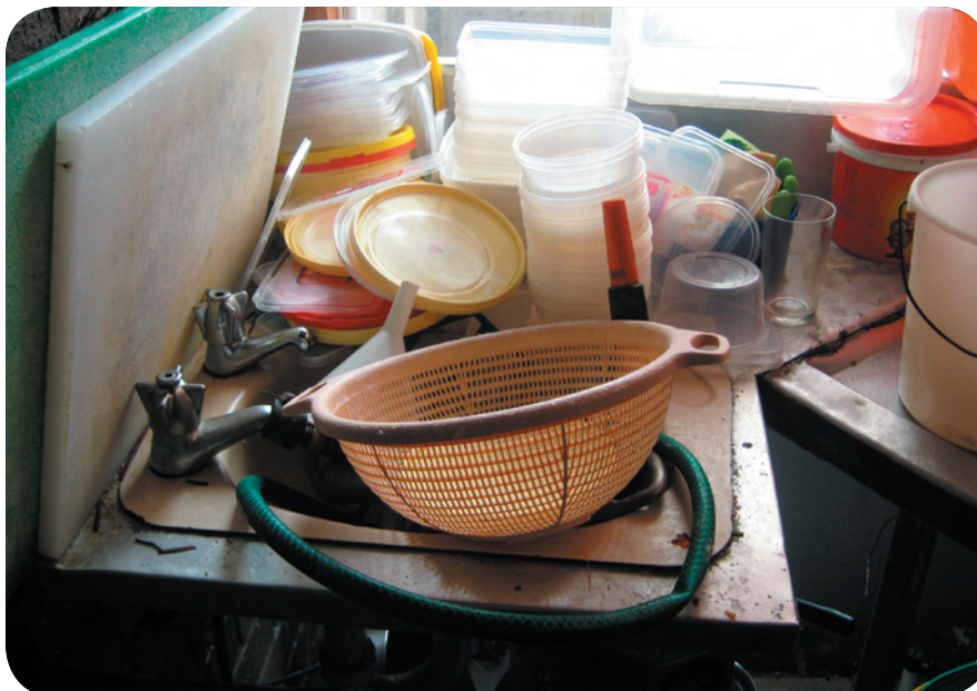
An obstructed hand wash basin
