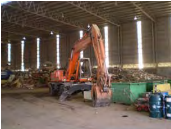
Resource Recovery Excavator
