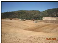
Progressive work to cap the site
