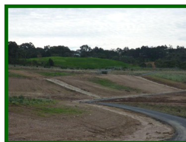
The reconstructed rock lined drains
