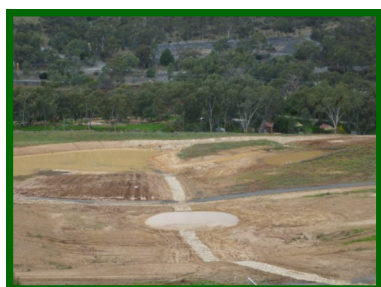
A new rock lined drain that was constructed to intercept runoff
