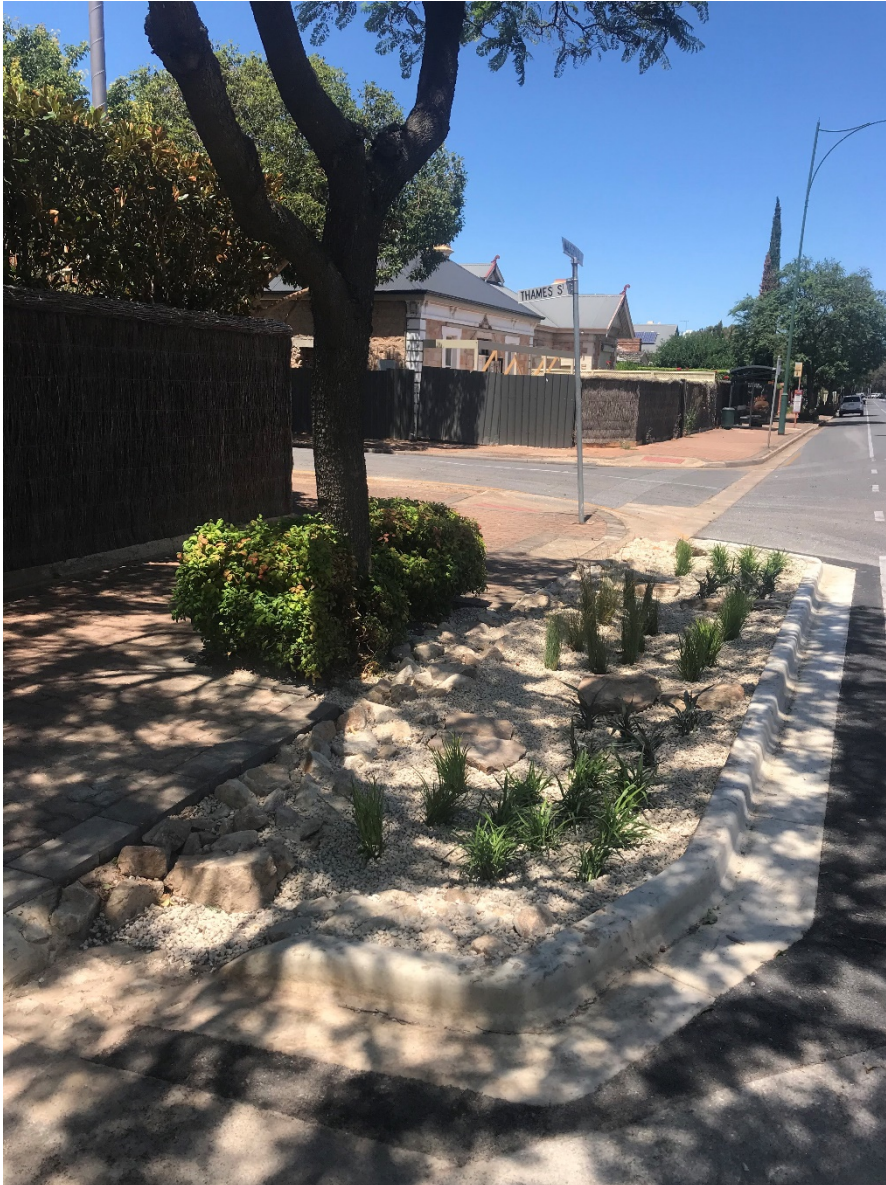
Newly planted out Water Sensitive Urban Design (WSUD) Rain Garden Walkerville Terrace, at the corner of Thames Street
