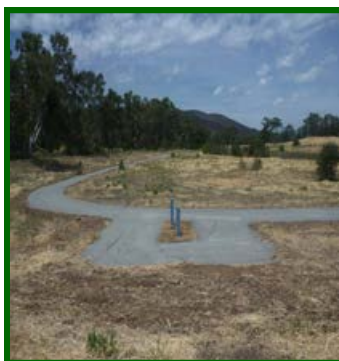
Monitoring Bore in the landfill
