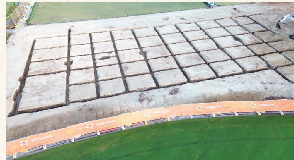
The Walkerville Bowling & Community Club site being prepared for the construction stage.
