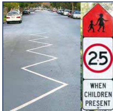
Review extent of School Zone and implement "25 km/h when children present" sign
