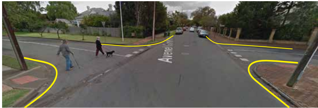
Avenel Gardens Road / Acacia Street / Glenfield Court looking north
