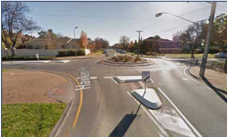
Example of a pedestrian connected roundabout Hawkers Road / Dutton Terrace in Medindie
