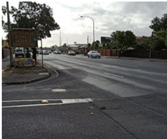
5:05 pm Queueing of westbound traffic minimal (looking east)
